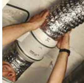
Connect the ducts.
