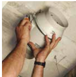
Place the impeller and motor assembly.
